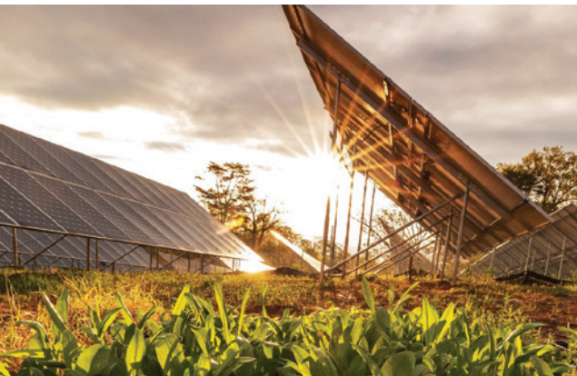
This Catholic Energies solar project in Washington, D.C., is part of an effort to show Catholic agencies that renewable energy can help their mission and their bottom line.
